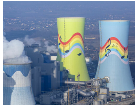
OPOLE POWER PLANT
