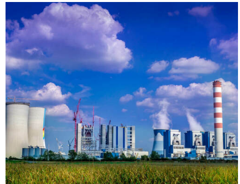
Power Plant Opole
