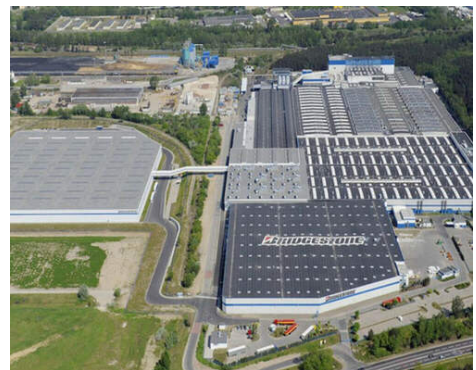
Production Hall Bridgestone, Poznań
